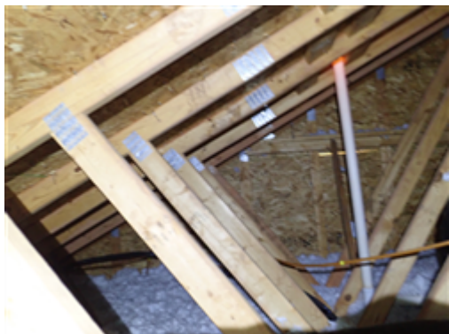
(A5 - 1.2 ) All Accessible Interior Areas
