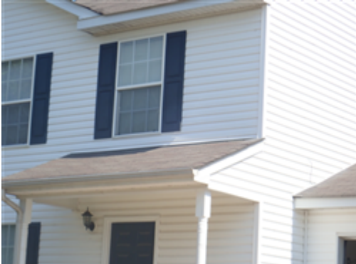
(C2 - 1) Main House Roofing: Drainage Systems (Descriptions):
