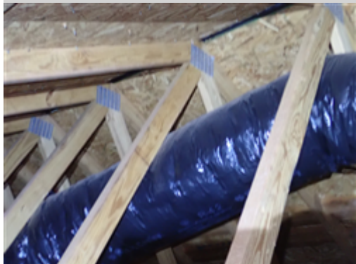
(A5 - 2 ) Structural: Ceiling Structure (Descriptions):
